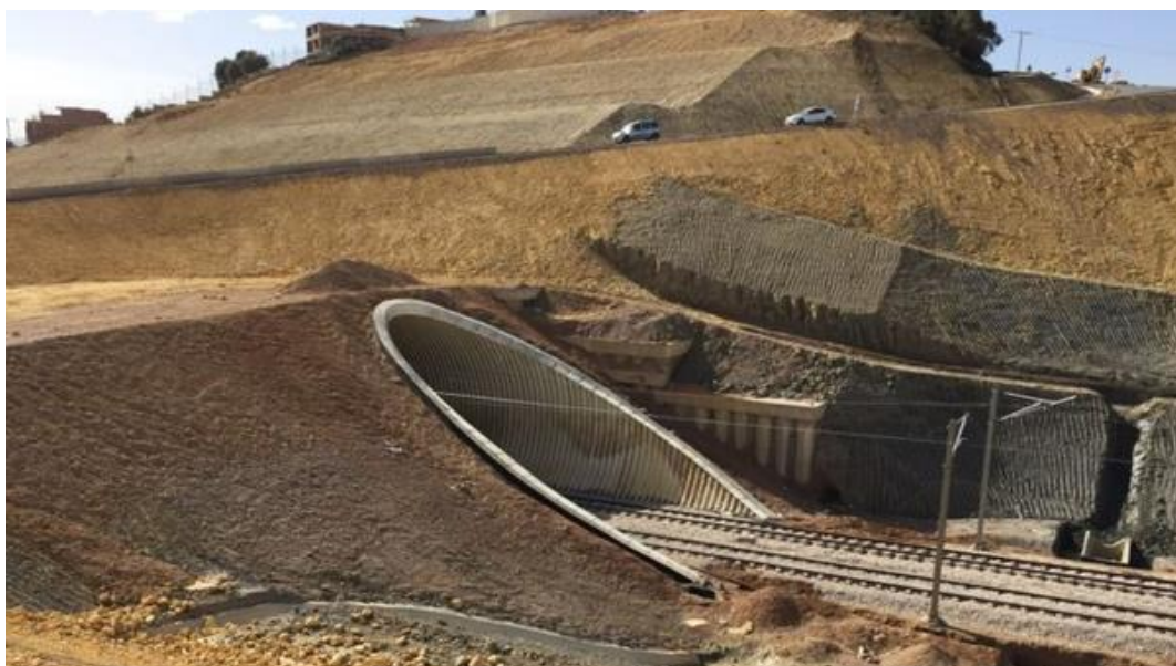
Figure 4. Railway tunnel Algeria (ViaCon Poland case study)
