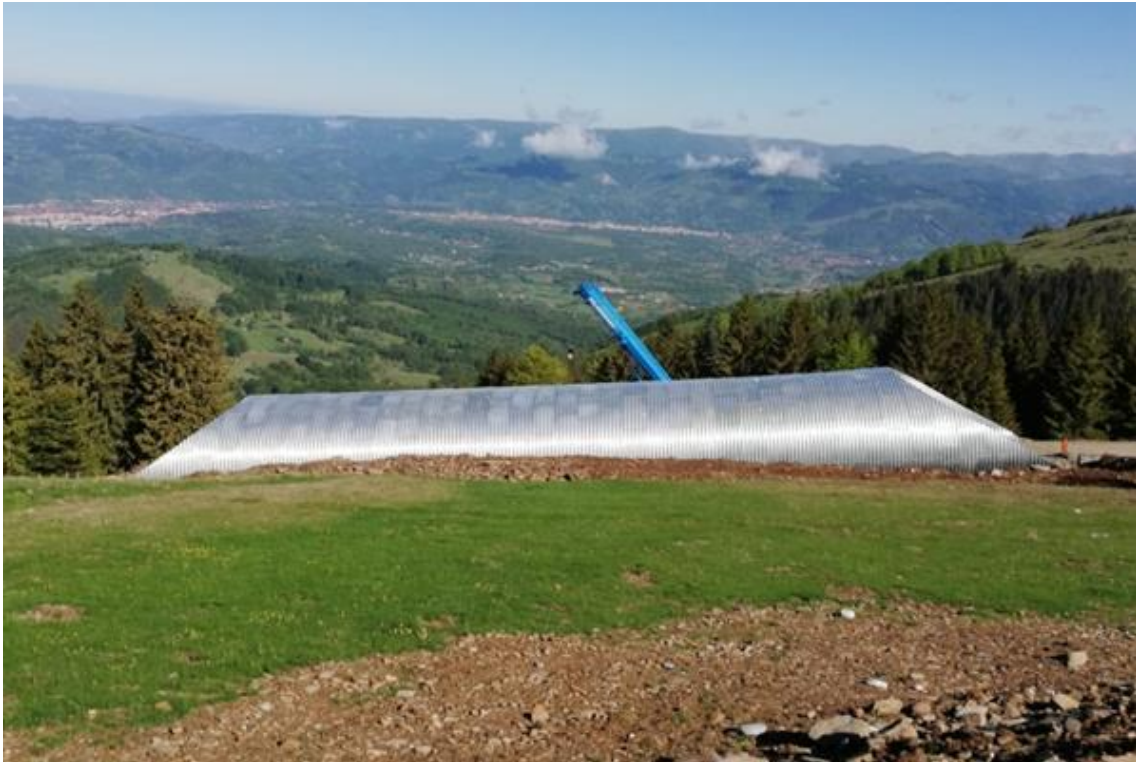
Figure 5. First steel tunnel (author photo)
