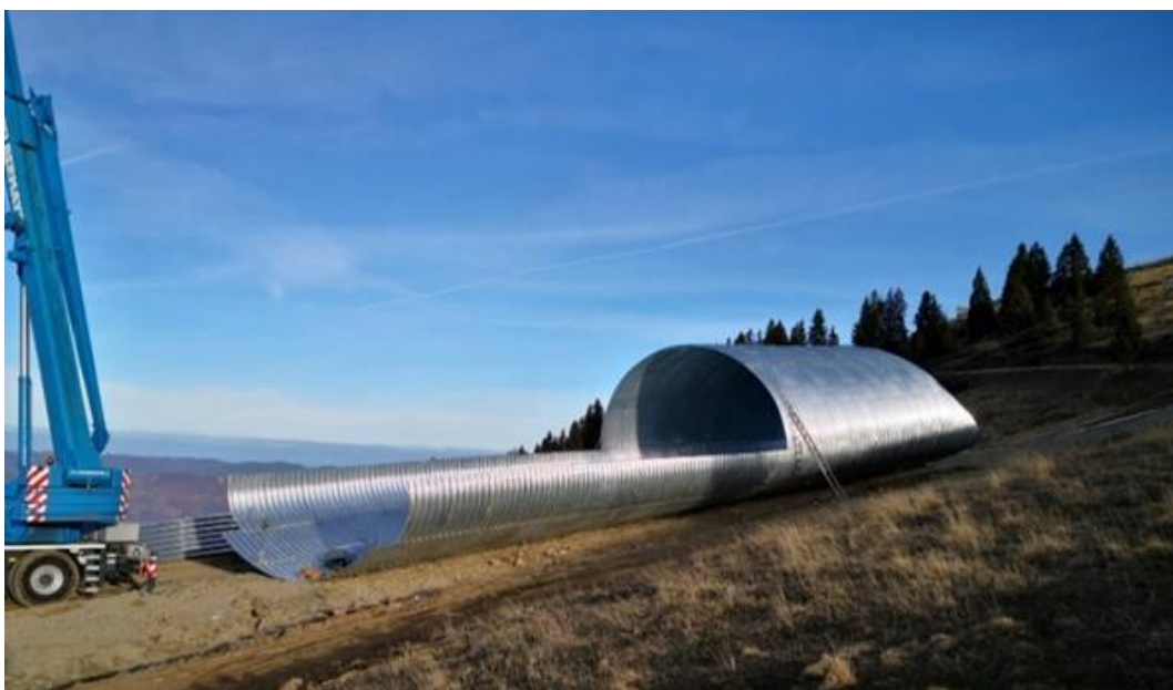
Figure 10. Assembly of side plates (author photo)
