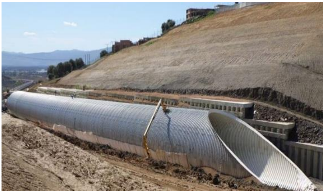
Figure 3. Railway tunnel Algeria (ViaCon Poland case study)
