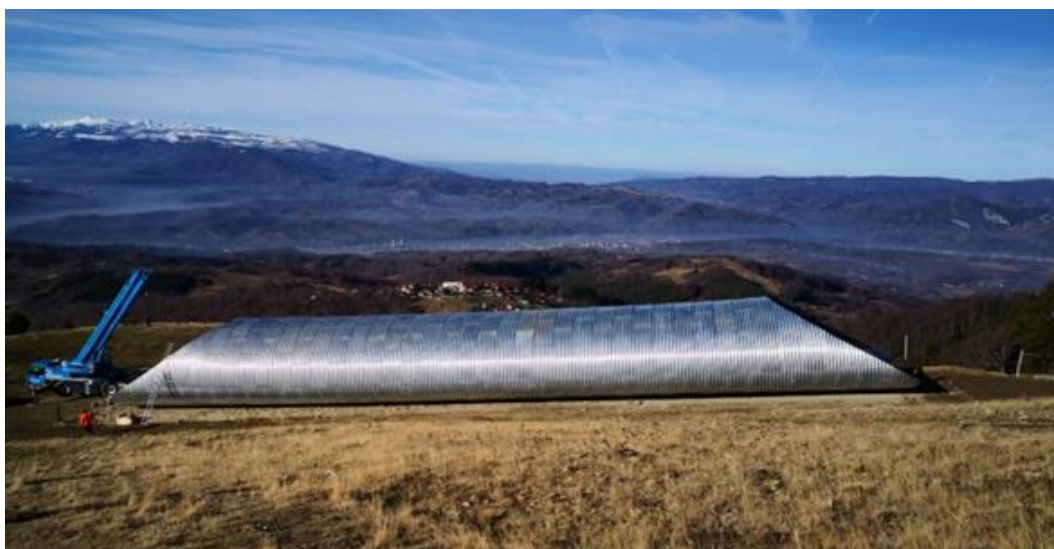
Figure 11. Assembly of top plates (author photo)
