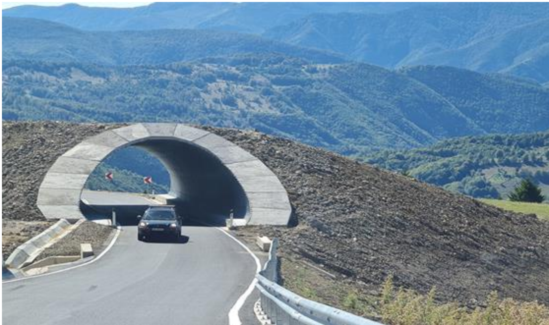
Figure 12. The final stage of the first tunnel (internet photo newspaper “Stirile Transilvaniei”)
