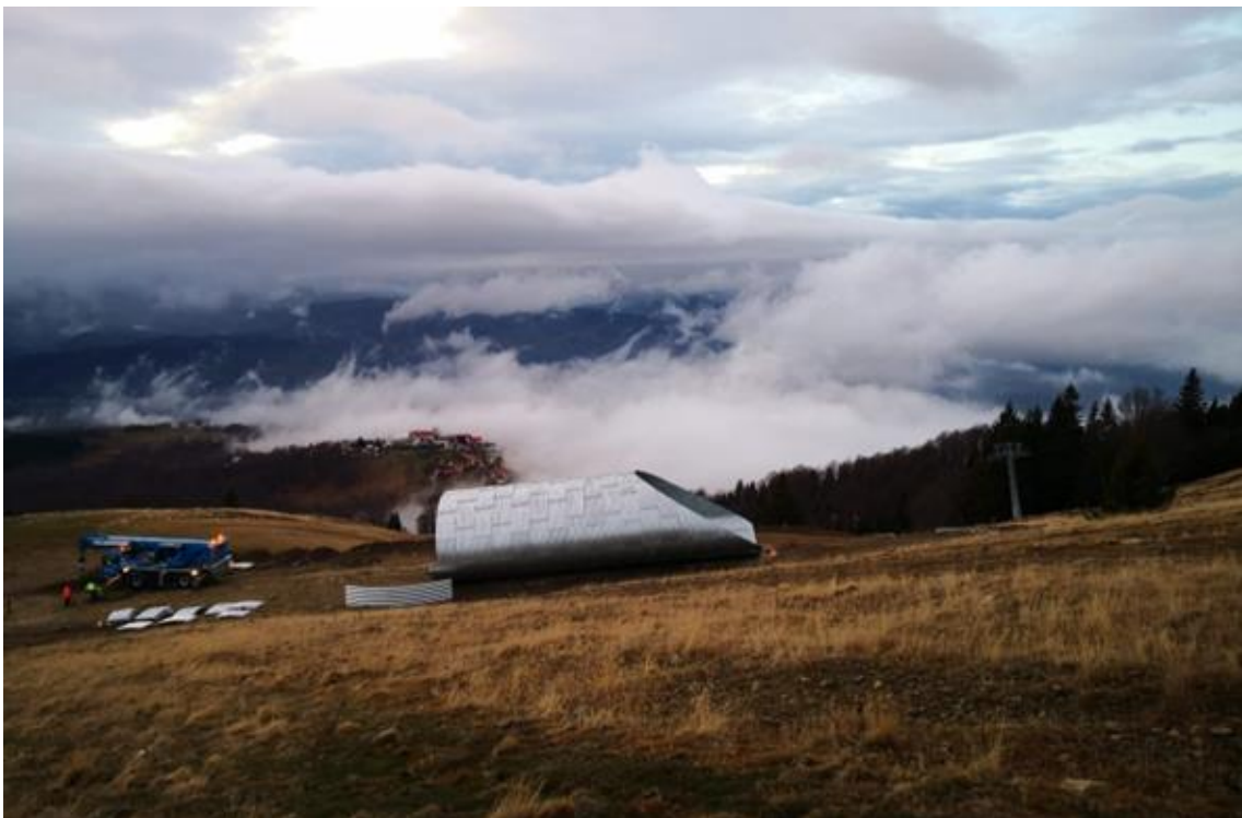
Figure 6. Second tunnel assembly in May 2020 (author photo)
