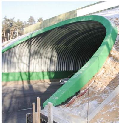
concrete headwall – bevelled end.
