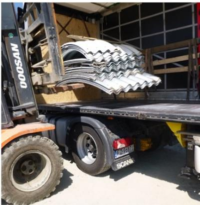
Unloading can be undertaken with a crane or an excavator and with straps. It is the contractor's responsibility to ensure that the unloading equipment has a suitable capacity to unload the materials safely. Small amounts of damage that may have occurred during transport and unloading may be repaired on the construction site after assembly. A repair paint kit is always delivered with each structure.
