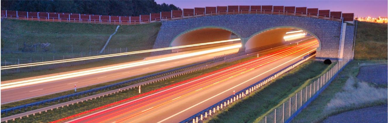
ViaCon ViaPlate & SuperCor® & UltraCor® are used mostly as buried flexible steel bridges & culverts, also called soil-steel structures. They are used for roads and railways infrastructure as well as for some industrial applications.
