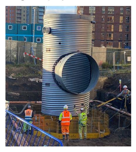
ViaCons One piece chambers, complete with flow regulators, pumps or even design with perforated pipe to be used as a soakaway. Tested and approved by Wrc, the chambers come complete with a 3 point lifting ring.
