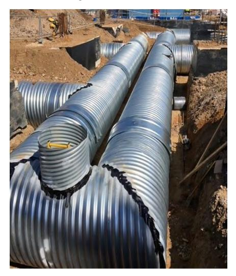
With this scheme in central London, we design the attenuation to zigzag in amongst the piles
